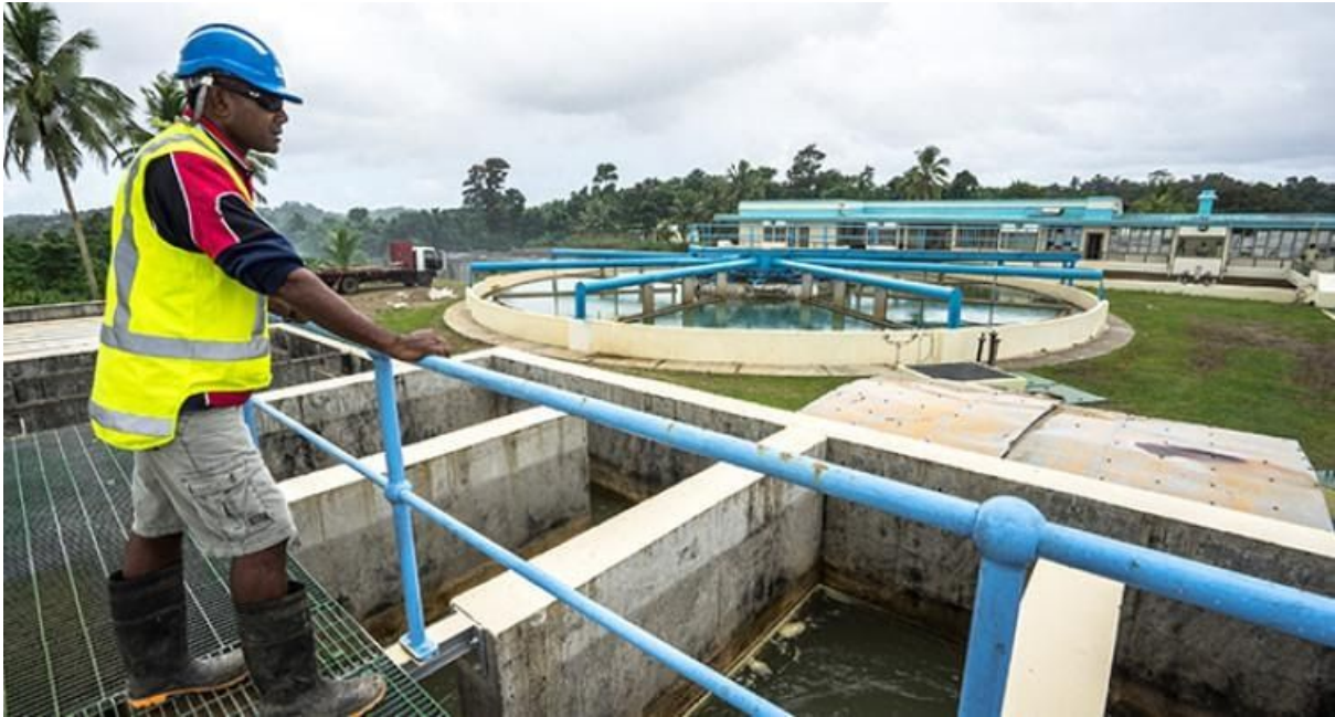
Figure 2: Waila Water Treatment Plant
