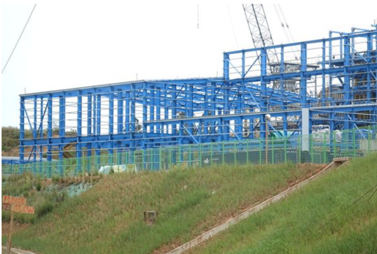
Figure 1: Construction of 10 MW biomass plant at Navutu, Sigatoka
